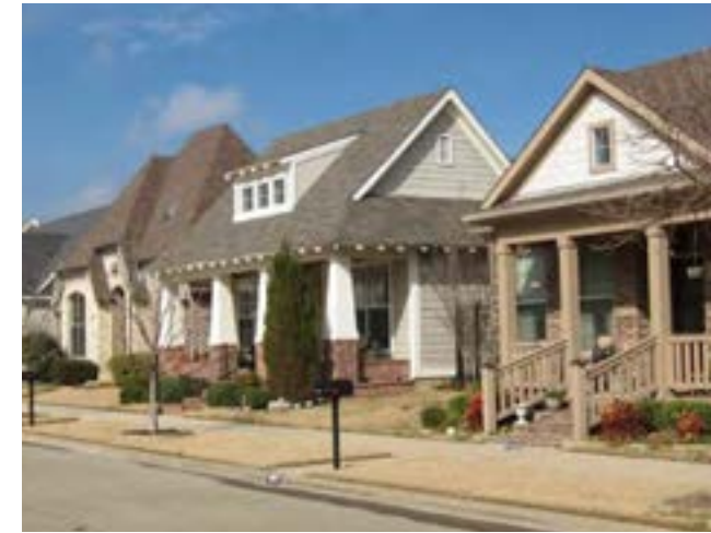
One to two story cottage homes
