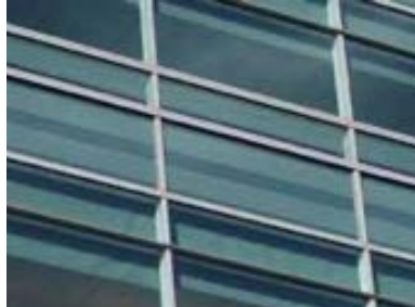
Glass Curtain Wall
