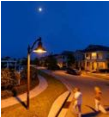
An example of a full cutoff fixture
