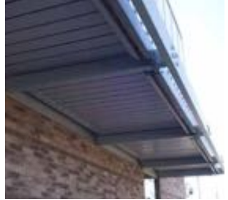
Soffit and Canopy
