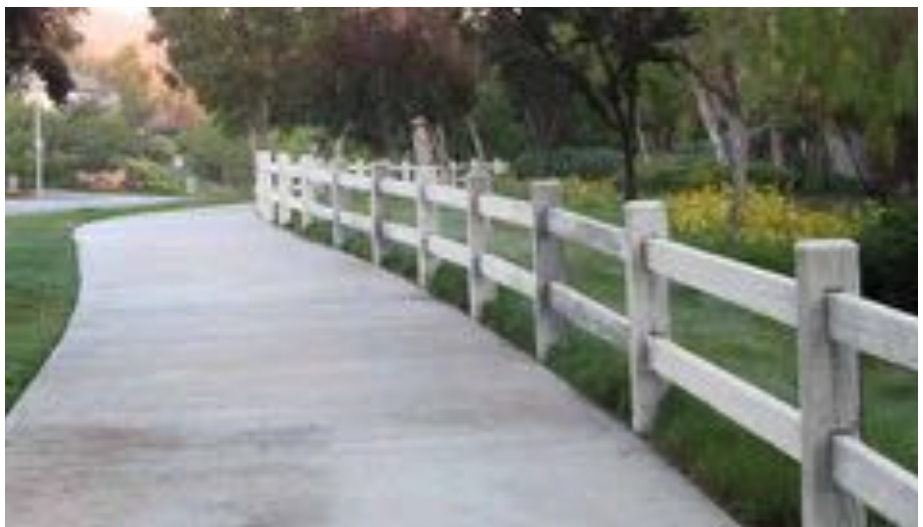
Composite "split-rail" fencing along greenway
