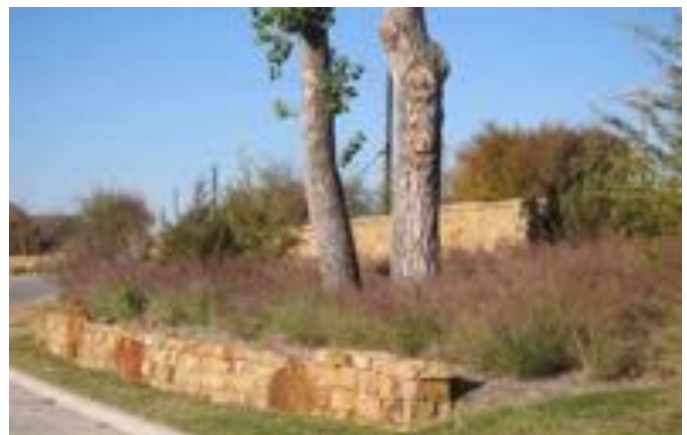
Terraced stone retaining walls
