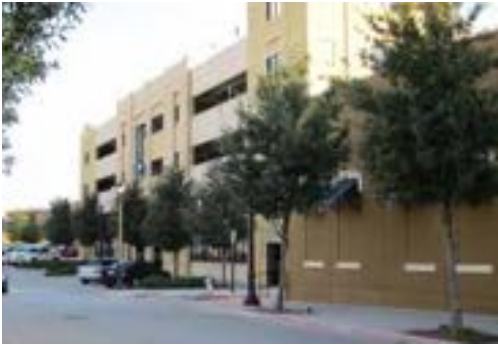
Trees lining parking structure and service drive
