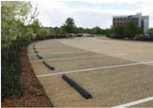
Surface parking lot with permeable pavement
