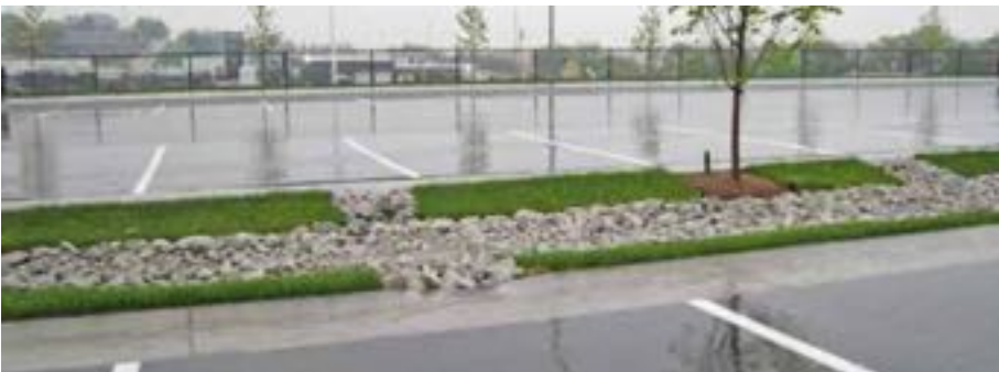
Bioswale within parking lot median
