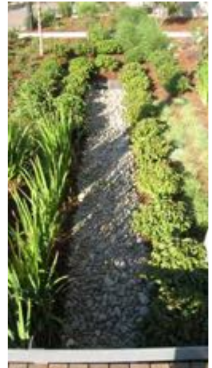
Dry creek bed and bioswale installation
