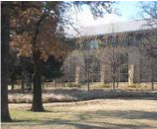
Expansive native landscape adjacent to an office building
