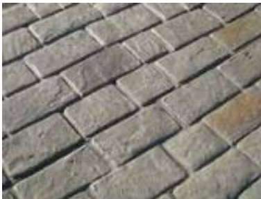
Stamped pattern in concrete
