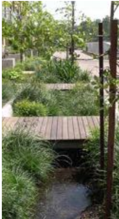
Stormwater planter in confined urban space
