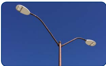
Newer LED street/parking lights like the ones pictured here are more energy-efficient than their older alternatives.
