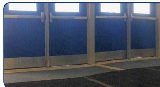
If light can enter through the envelope of these UNK doors, then heated and conditioned air can pass through the envelope, as well, resulting in wasted energy.
