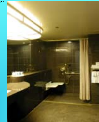
Figure 3. Safety guidelines for a shower include slip-resistant flooring, roll-in accessibility, seating in shower, hand-held shower head, grab bars and lighting in shower.
