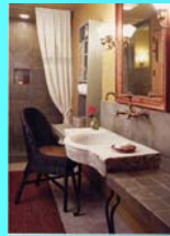
Figure 1. When a bathroom sink is attached directly to wall it allows for knee space.
